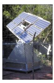
A Remote Area Power Supply (RAPS) system is installed. The system used is a commercially available system (Pyramid Power). This includes a solar tracking array of Photo Voltaic (PV) cells, an inverter, a battery bank and a backup generator. The batteries and control system are mounted in a pyramid shaped storage box underneath the panels. The backup generator is rarely required.
