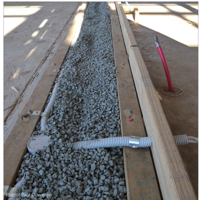
Another kind of base plate with a lower profile and no crosspieces. Note early placement of conduit to accept wiring.
