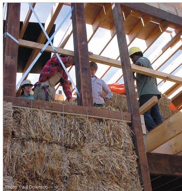
The middle plate and compression wires can be seen in this detail of a timber framed, three storey strawbale townhouse.
