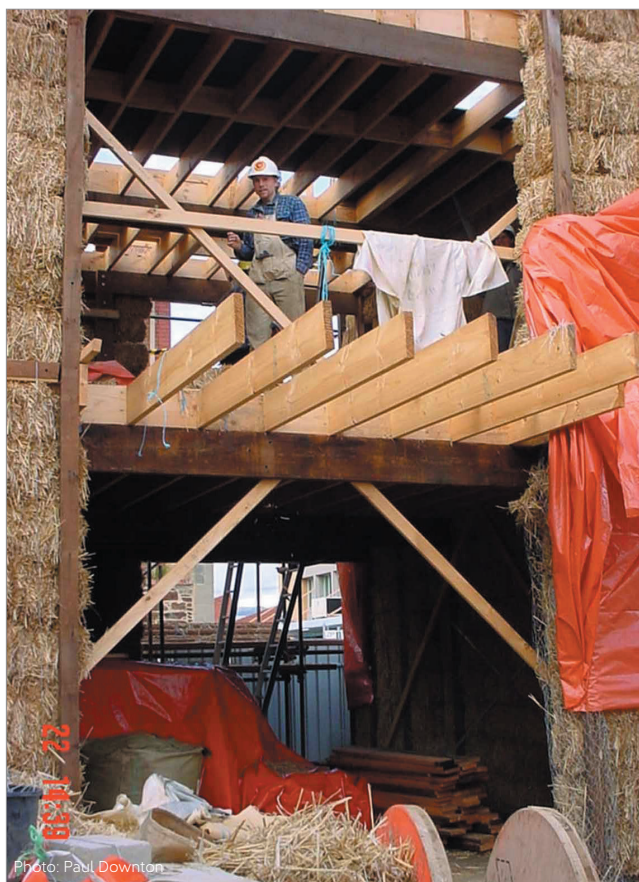
The use of frames makes almost any kind of opening possible in strawbale construction.
