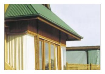
Above, standard 2100 high doors are shaded by a 1000 eave (including gutter) set 300 above the head. Note the sun angle at midday in mid winter is above the glass line. This configuration provides full shading to glass from late October to late February at latitude 35°S (near Canberra) and is appropriate for a higher altitude cool climate winter.
