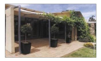
**Pergolas** covered with deciduous vines provide self adjusting seasonal shading. A 500mm gap between the wall and planted screens should be left for ventilation and cooling. Vines on walls (where appropriate) can also provide summer insulation to all orientations. Evergreen vines block winter sun and should only be used in tropical climates.
