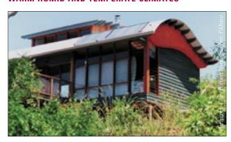
**Provide** passive solar shading to all north facing openings, using shade structures or correctly sized eaves
