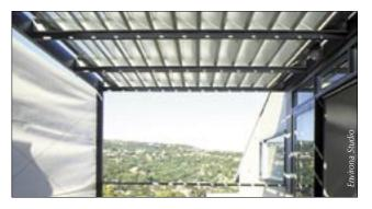
**Adjustable shading** appropriate for northern elevations includes adjustable awnings or horizontal louvre systems above glazing, and removable shadecloth over pergolas or sails. Shadecloth is a particularly flexible and low cost solution.
